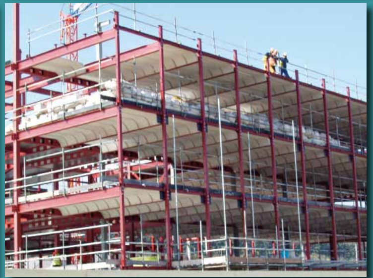
Photographs of storage and installation of profiled slabs supplied to the new Welsh Assembly Building at Aberystwyth.
