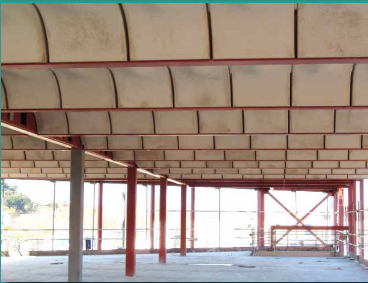
Photographs of storage and installation of profiled slabs supplied to the new Welsh Assembly Building at Aberystwyth.
